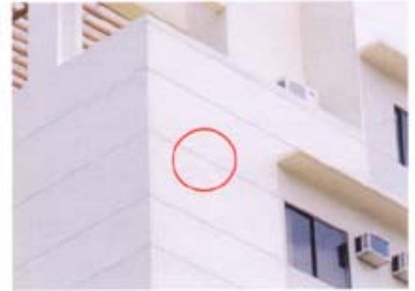
GV3 PLASTERING GROOVE LINE 15MM PLGI.B01 -10X15MM
